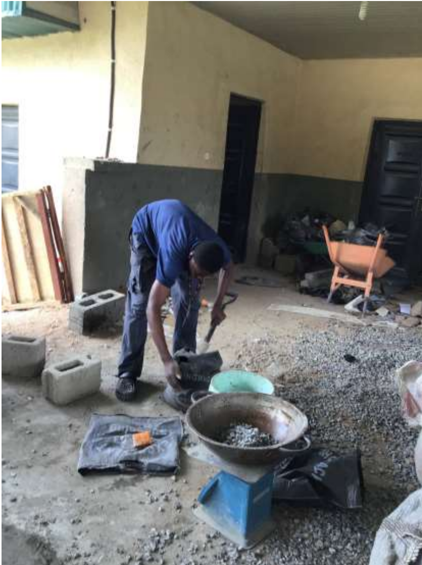
Fig: weigh and mixing of concrete samples
