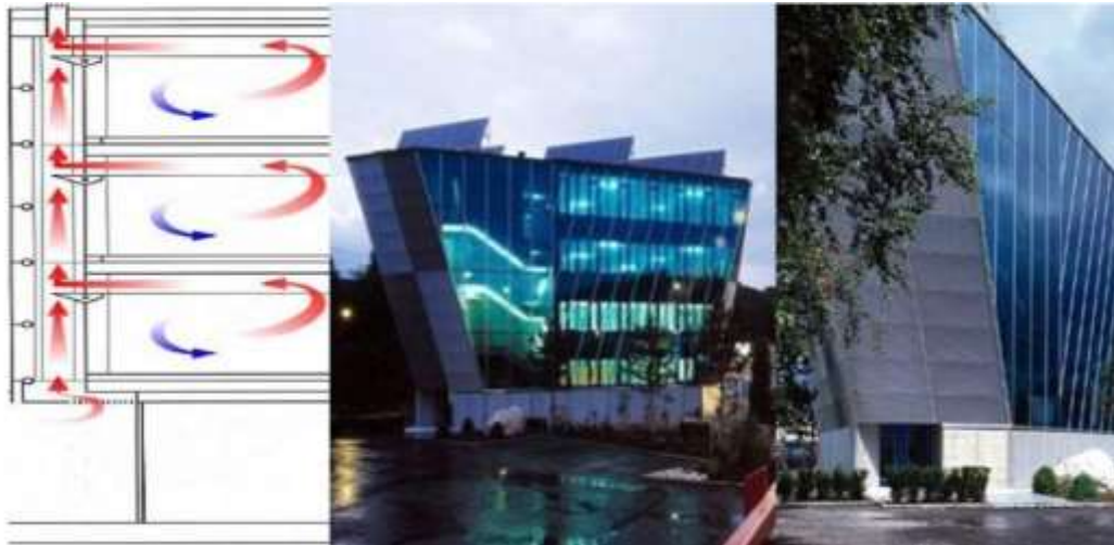
Fig. 5: Extract Air DSF Figs. 6 & 7: Bürogebäude Felbermayr, Salzburg, Austria. Source: T Boake UW Source: www.architecten.at
