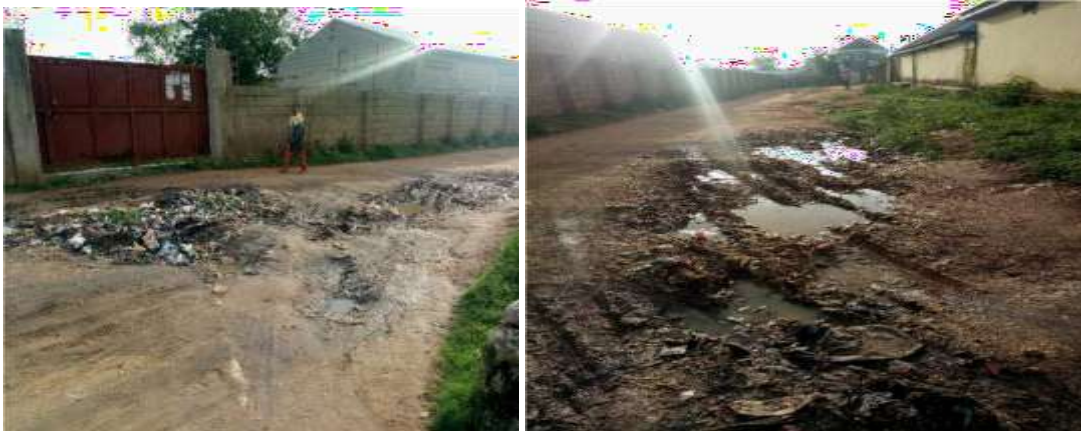
A Street without drainage and official dump site, water lodge eroded road littered with refuse.
