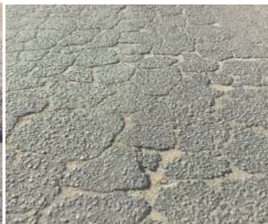
Alligator Cracking
