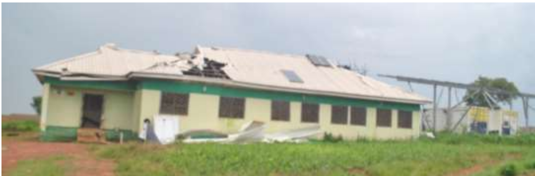
Image 5: A roof affected by wind.
