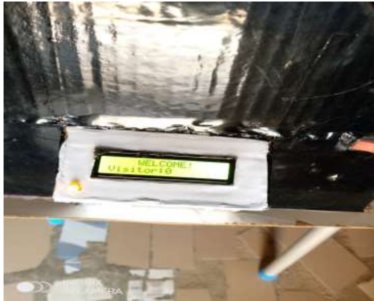
Fig 4. System Assembling and Casing of Automatic Room light Controller with Visitor counter
