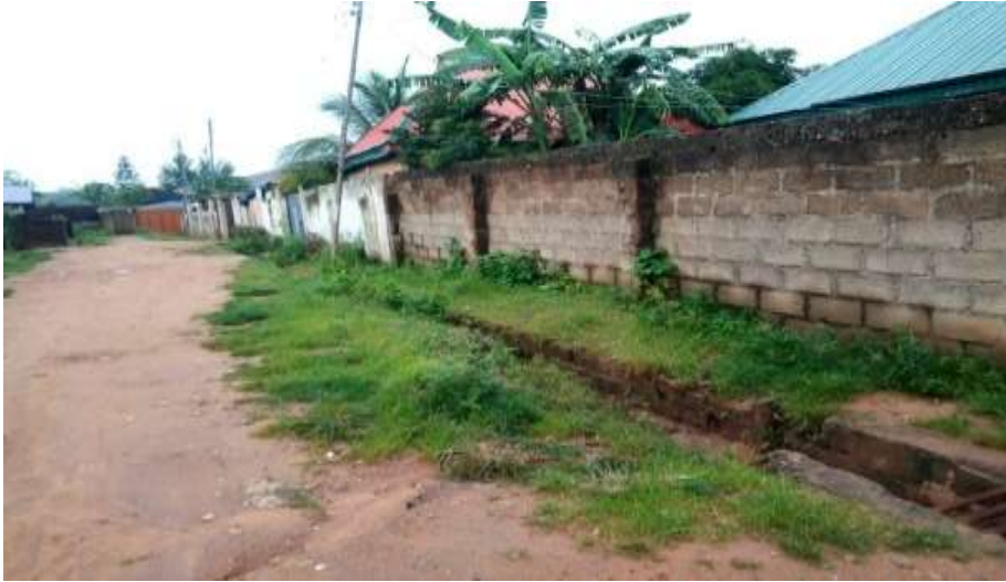
Plate 3: Building Line and Unkept Drainages
