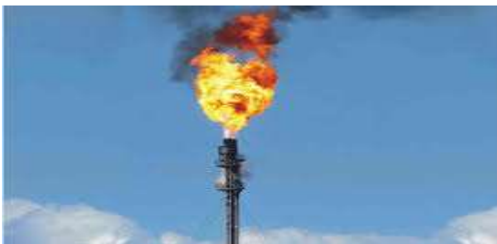
Figure 1 Gas flare facility (Source, Gas flare images 2019)
