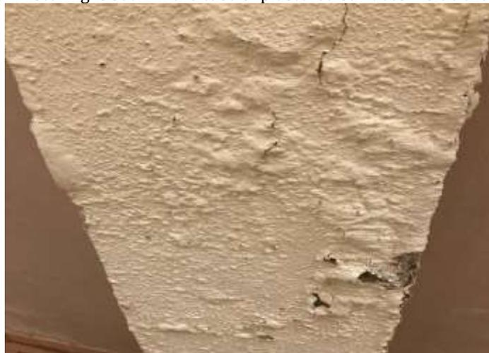
Figure 7 showing Wall with Blistering of Plastered surface
